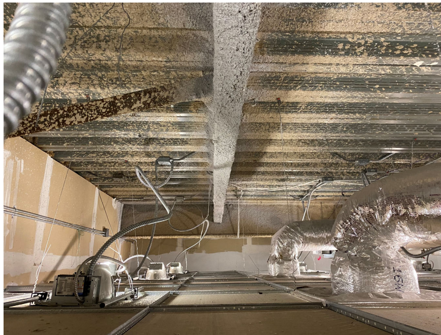
Photo 2: View of typical above-ceiling finishes at Hofheimer Hall. No samples collected were determined to contain asbestos.
