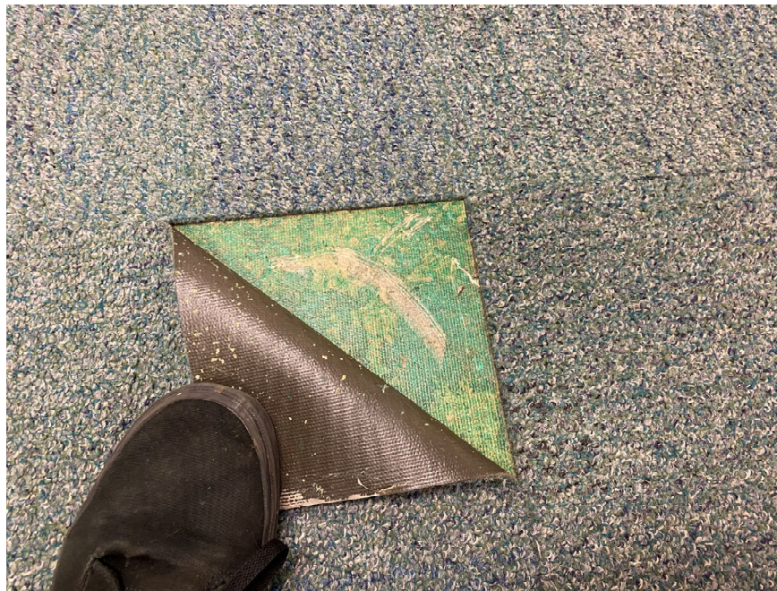
Photo 6: In areas with carpet, carpet mastic was observed under carpet squares. The material was determined not to be asbestos-containing.
